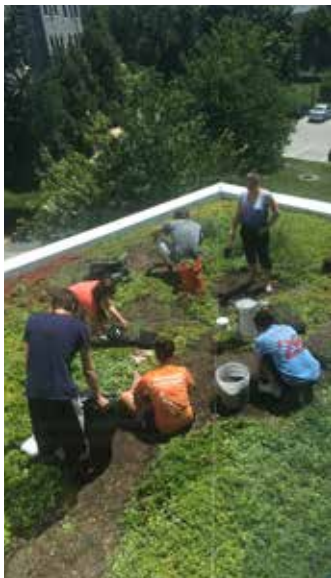
The green roof on the Center for Engineering Education and Research (CEER) is just one of several stormwater research and demonstration sites on campus.
