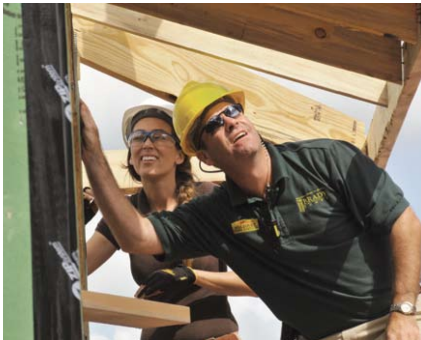
Bob works on the house with “Extreme Makeover: Home Edition” home designer and host Didiayer Snyder.
