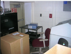
Ensure boxes/ materials are not blocking egress routes
