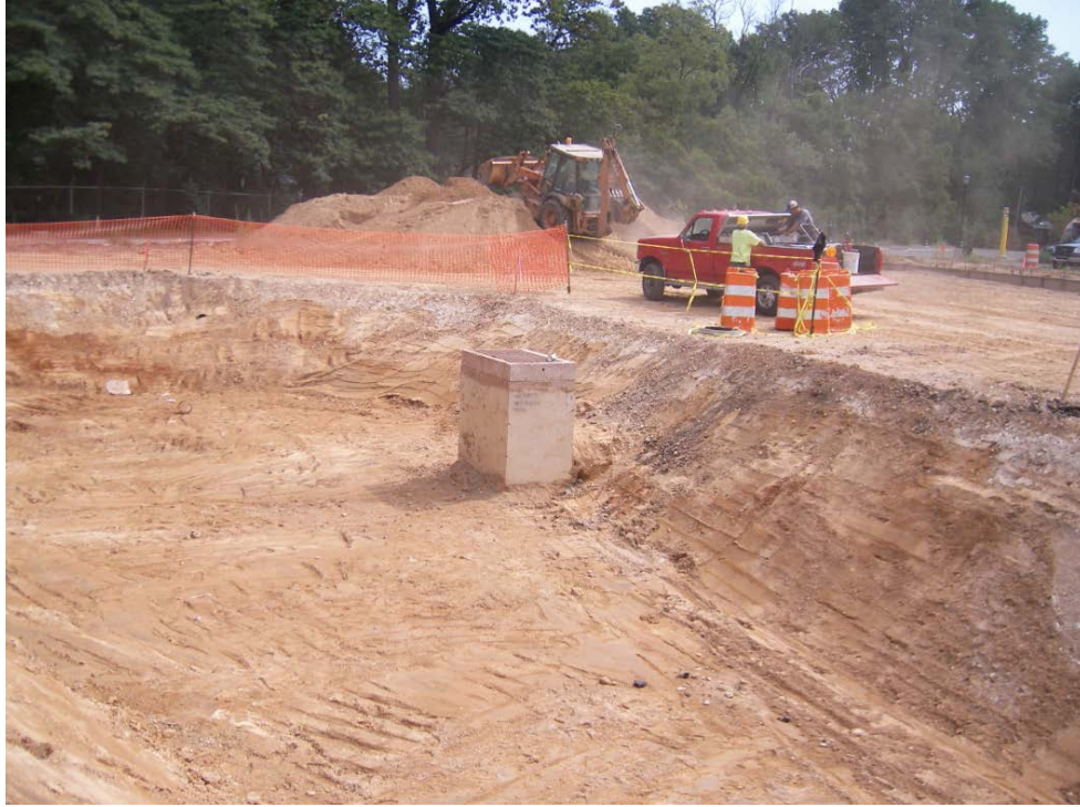
Figure 3.28 Construction of the PTI (photograph courtesy of Villanova Urban Stormwater Partnership)
