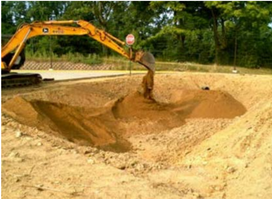
Figure 3.49 Soil mix being placed at the BTI in 2001 (Prokop)
