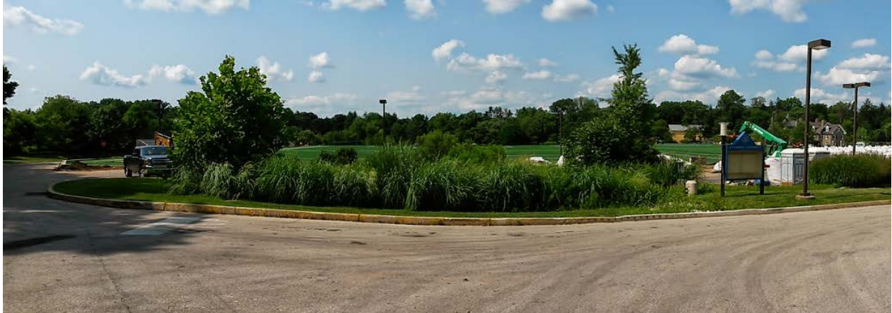
Figure 1.5 The Bioinfiltration Traffic Island (photograph courtesy of Villanova Urban Stormwater Partnership)
