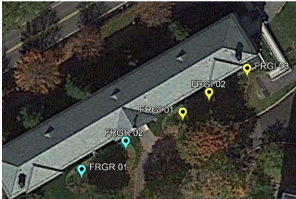
Figure 6.6 Infiltration test locations at the FRG
