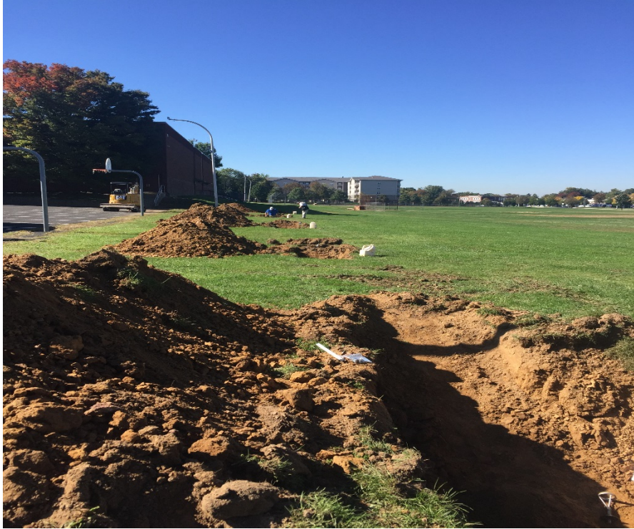
Figure 6.8 Test pits dug at the Upper Moreland site
