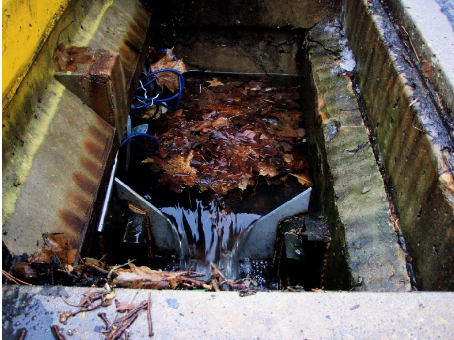
Figure 3.59 Leaves in the outlet box at the BTI (photograph courtesy of Villanova Urban Stormwater Partnership)
