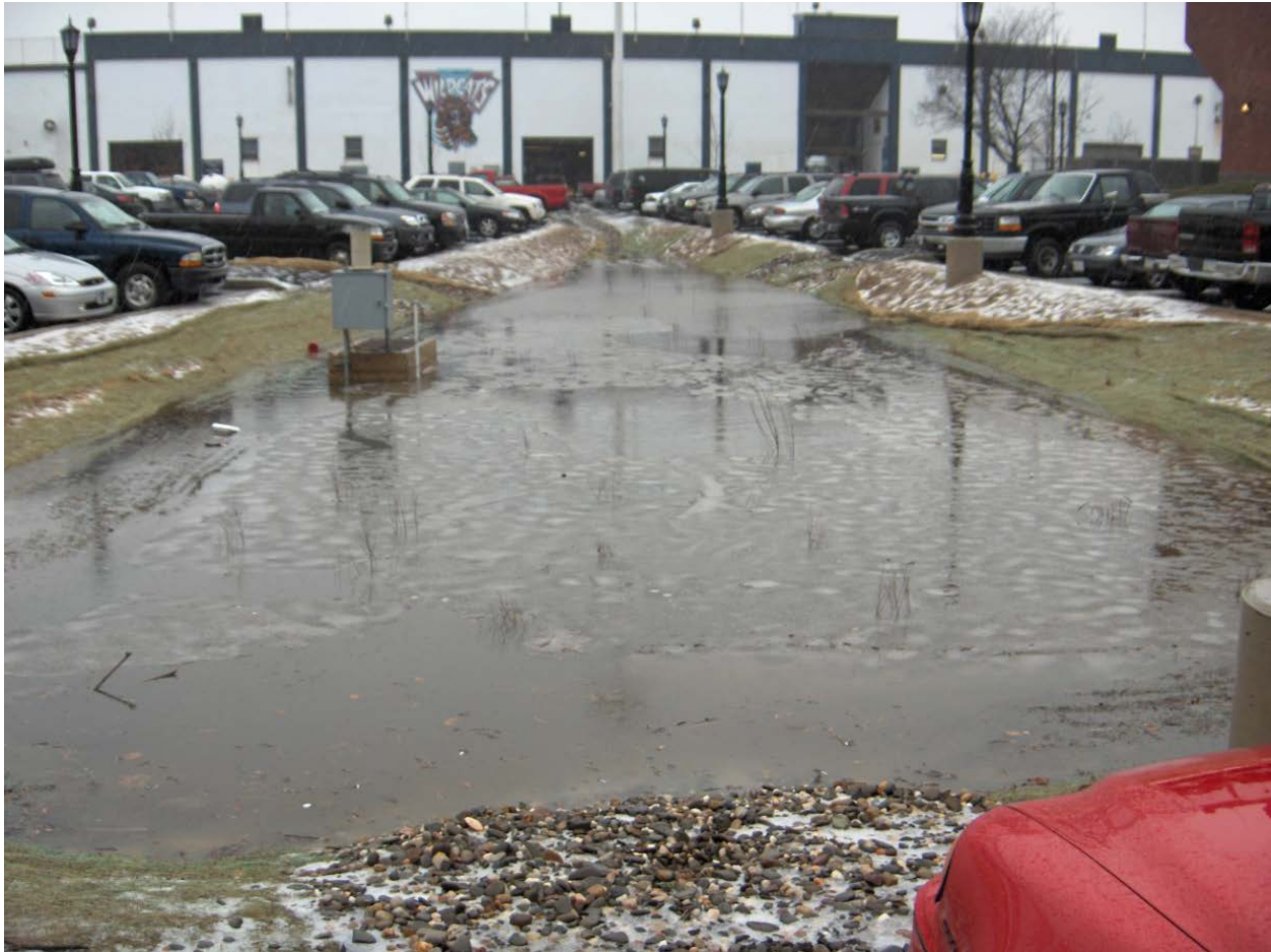
Figure 3.40 Ponding at the PTI after a rain event (photograph courtesy of Villanova Urban Stormwater Partnership)
