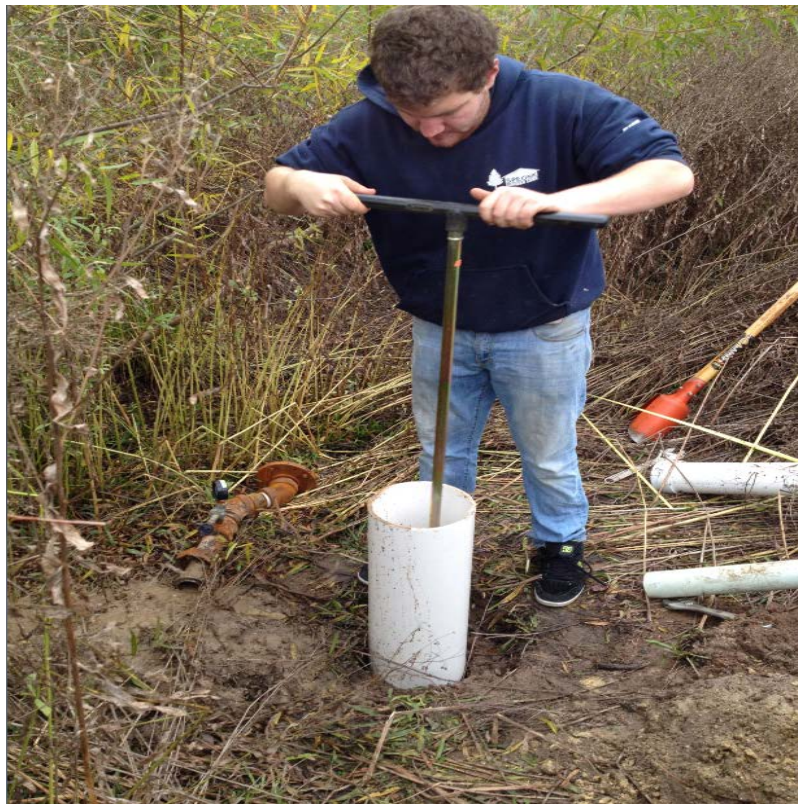
Figure 3.36 Monitoring well installation at the PTI
