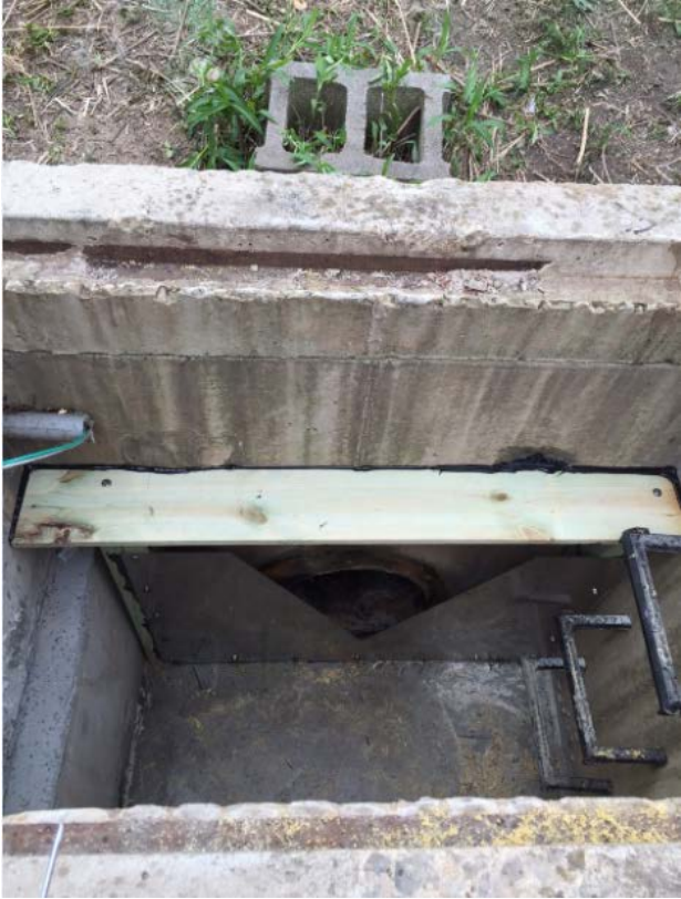
Figure 3.34 Concrete box repairs and new 60° V-notch weir at the PTI
