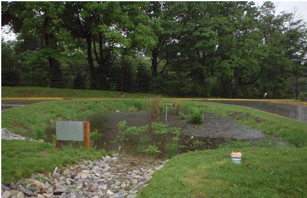
Figure 1.9 The BTI ponded during a rain event (photograph courtesy of Villanova Urban Stormwater Partnership)
