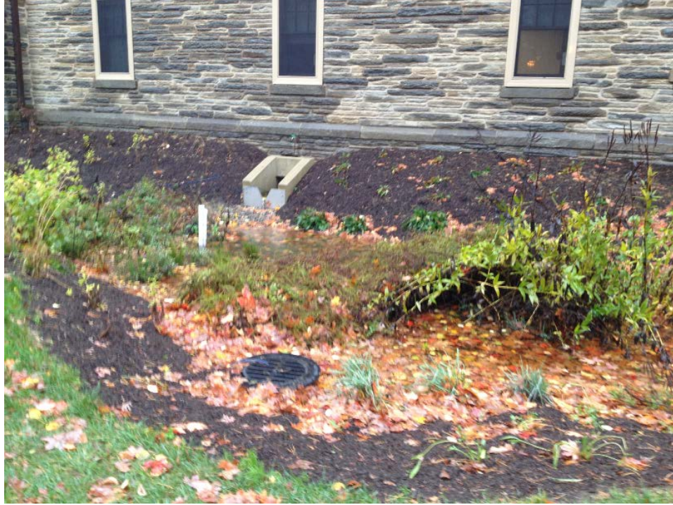
Figure 3.12 Leaves in the FRGR at Fedigan Hall (photograph courtesy of Villanova Urban Stormwater Partnership)
