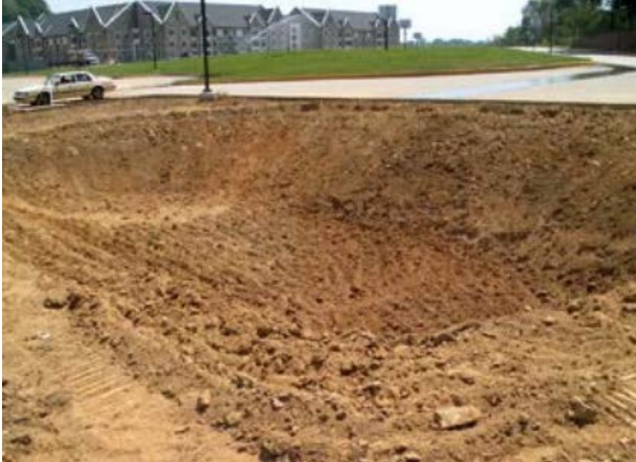
Figure 3.48 Construction at the BTI in 2001 (Prokop 2003)
