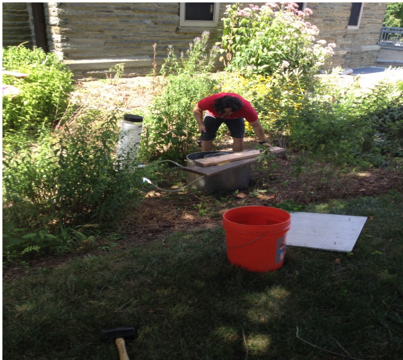
Figure 6.4 FRGI-02 being installed at the FRGI
