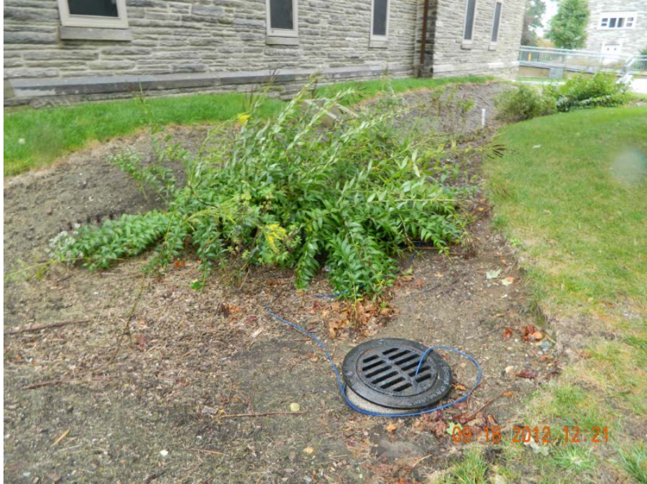
Figure 3.3 The completed FRGI at Fedigan Hall (photograph courtesy of Villanova Urban Stormwater Partnership)
