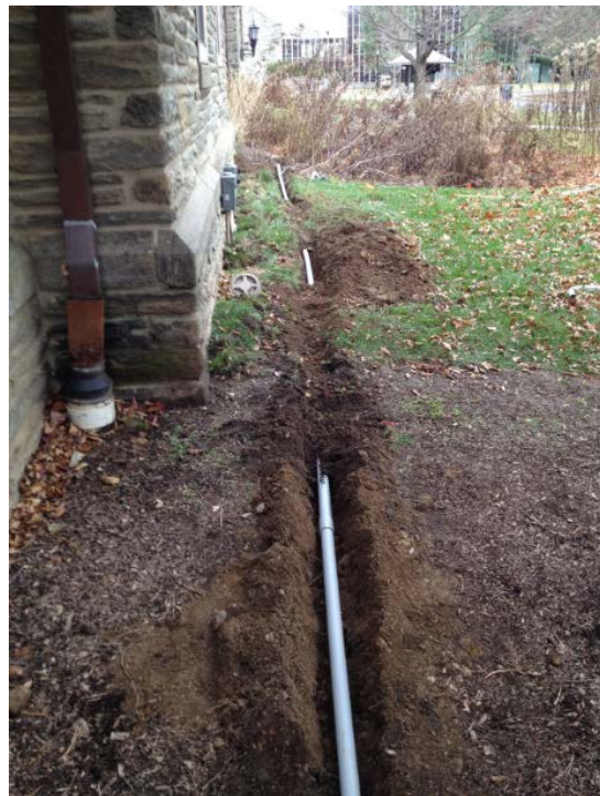
Figure 3.7 Conduit installation at the FRGR
