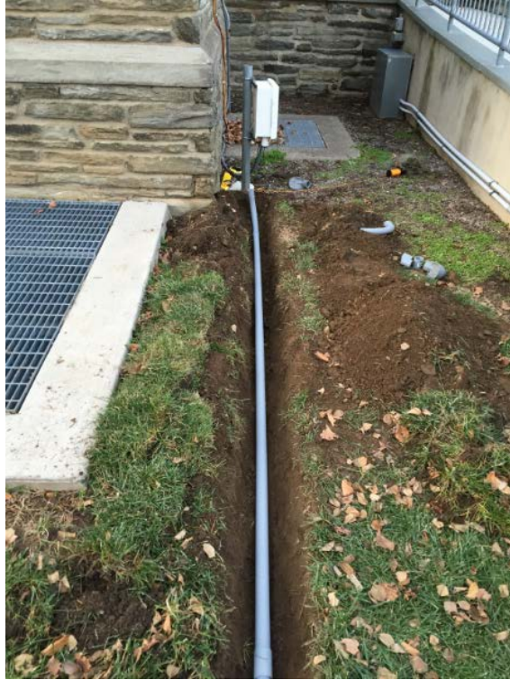
Figure 3.6 Conduit installation at the FRGI
