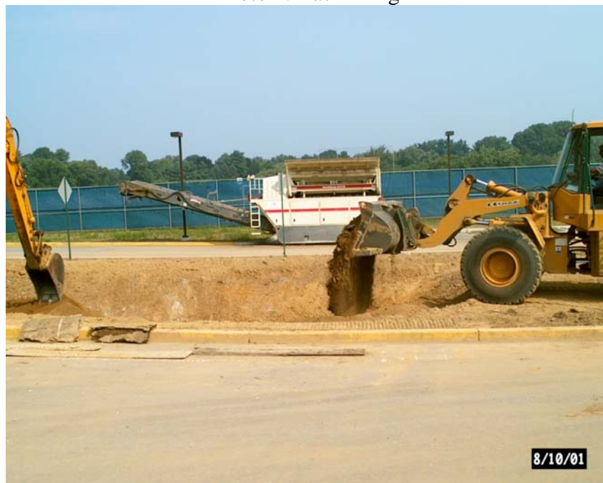
Photo 4: Backfilling
