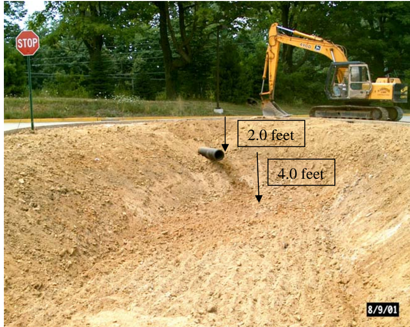
Photo 3: Storm drain inlet – overflow installation
