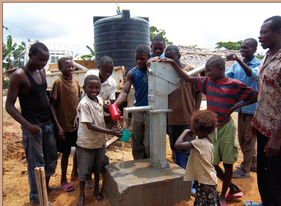
An Afridev hand pump is installed and ready for operation following the drilling of a well to nearly 200 feet in Yanongi, 22 miles south of Kisangani in the Orientale Province in the Democratic Republic of the Congo on April 22, 2011. Photo courtesy Congo Frontline Missions.
