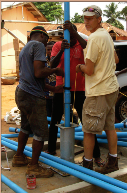
David Powell, CWD/PI, helps with a hand pump installation in the Volta Region of Ghana.
