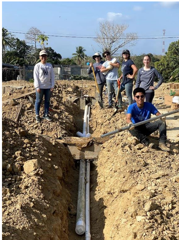
10 - Installing pipes for the Community Parish Center.
