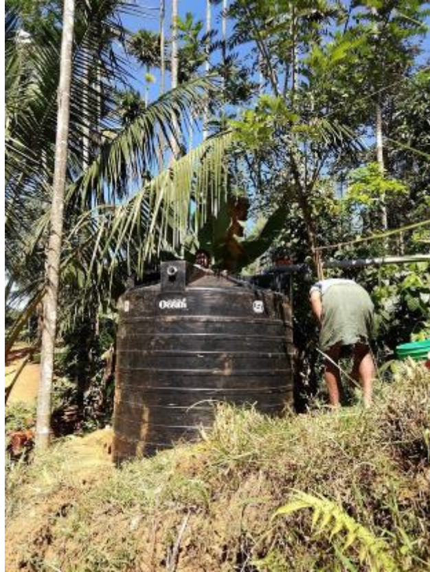
19 - India: Image of a storage tank we helped install that will collect water from the rooftop of the users house.
