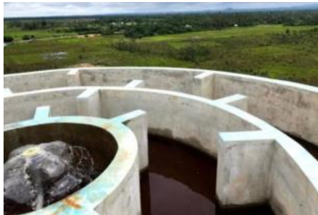
8 - Photo of the water tank the treatment review was completed for.
