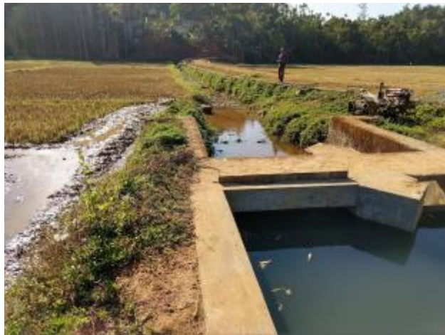
17 - India: Photo of irrigation practices used by a local tribe. They implement a series of trench distribution systems.
