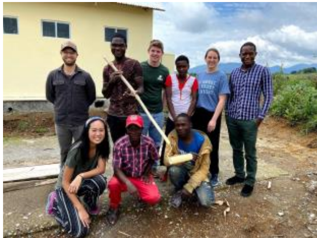
22 - Tanzania: Members of the Villanova team with local entrepreneurs hired by CRS to construct latrines for a local school.
