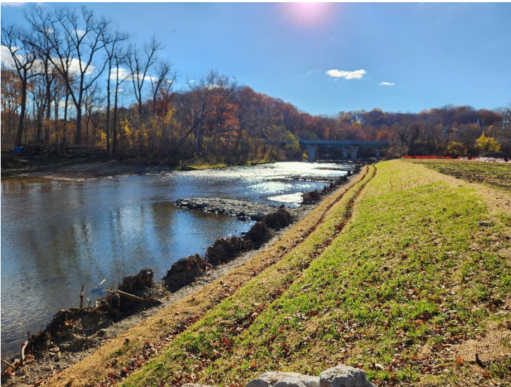
Figure 2. Constructed Engineered log bank protection and bendways weirs
