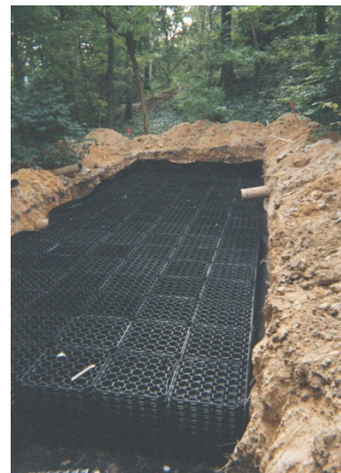
Figure 2 – Construction Photo of Rainstore System
