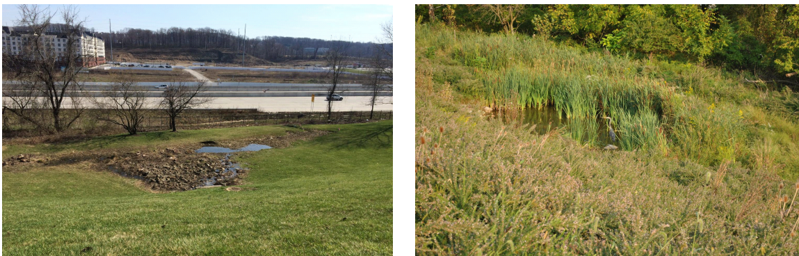
Figure 2. Existing Basin Outfall Scour and Restored Condition
