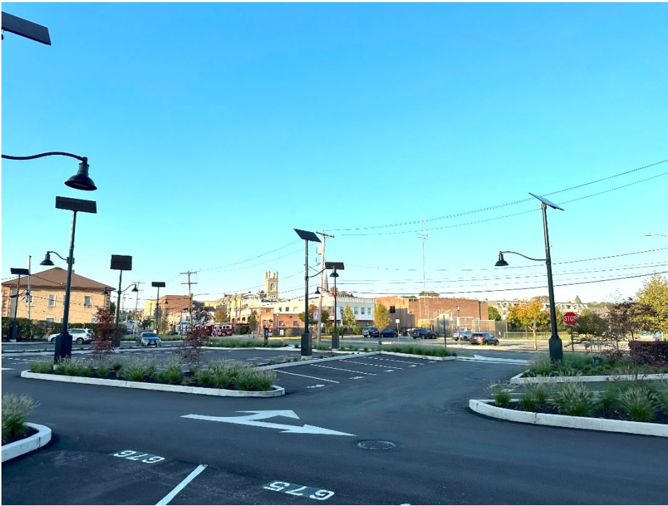
Figure 3. Photo of constructed improved parking lot.
