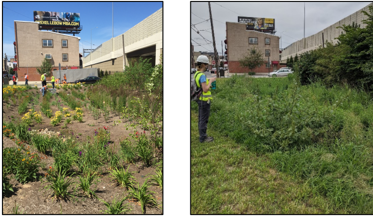
Figure 1. A basin along I-95 whose plant palette was not salt tolerant. Images were taken in 2017 (left) and 2020 (right).
