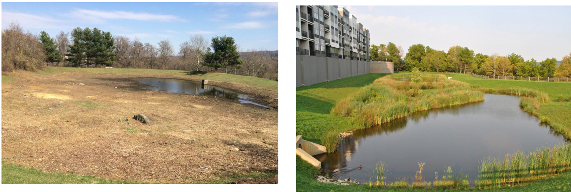
Figure 1. Existing Extended Detention Basin and Retrofitted Constructed Wetland
