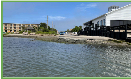
Figure 1. Straughan project site at Dagsworthy Street, Dewey Beach, DE
