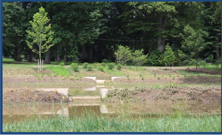
Figure 1. Substantially Complete Sloping Wetland System following 4-inches of rainfall in less than 4 hours on July 12, 2021 (~100-year storm).
