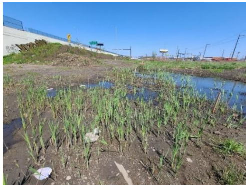
Figure 1. Site of a stormwater basin which encountered a high groundwater table prior to construction.
