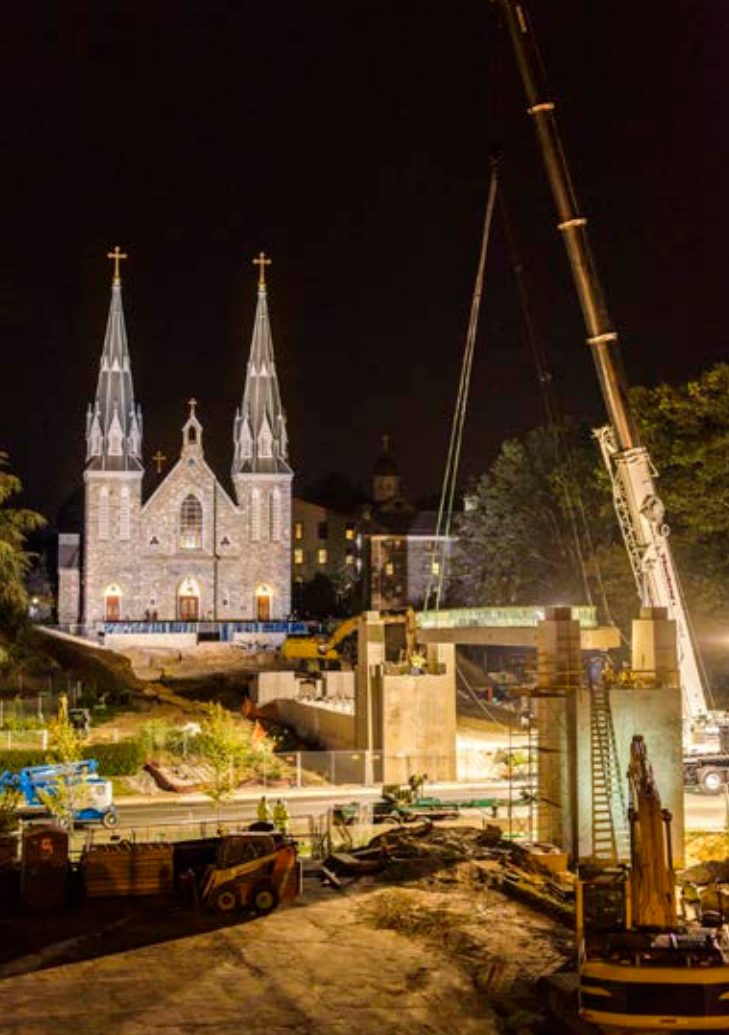
The pedestrian bridge in front of St. Thomas of Villanova Church takes shape as workers lower the center beam into position.
