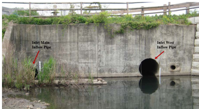
Figure 1-3: Inflow Pipes
