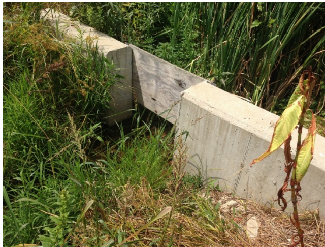
Figure 1-7: Adjustable Sluice Gate
