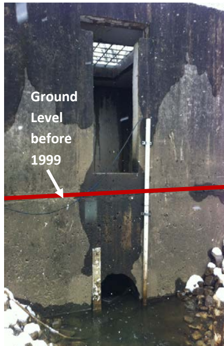
Figure 1-4: Outlet Structure
