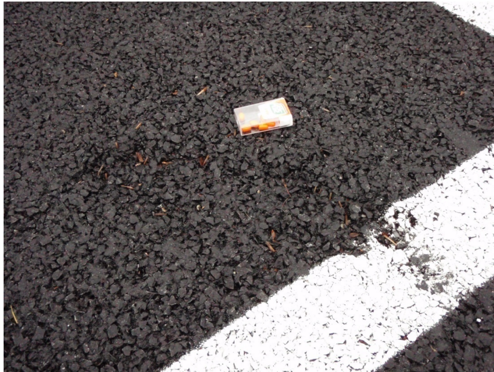
Figure 5-3 Depression in Porous Asphalt
