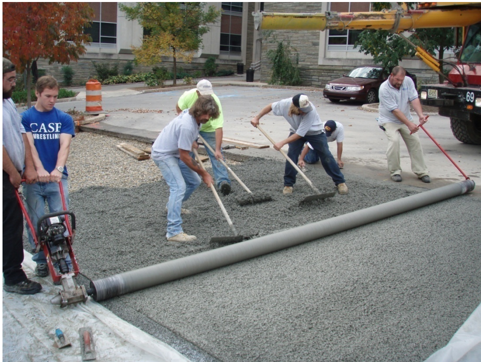
Figure 4-5 Pervious Concrete Installation Using Roller Screed
