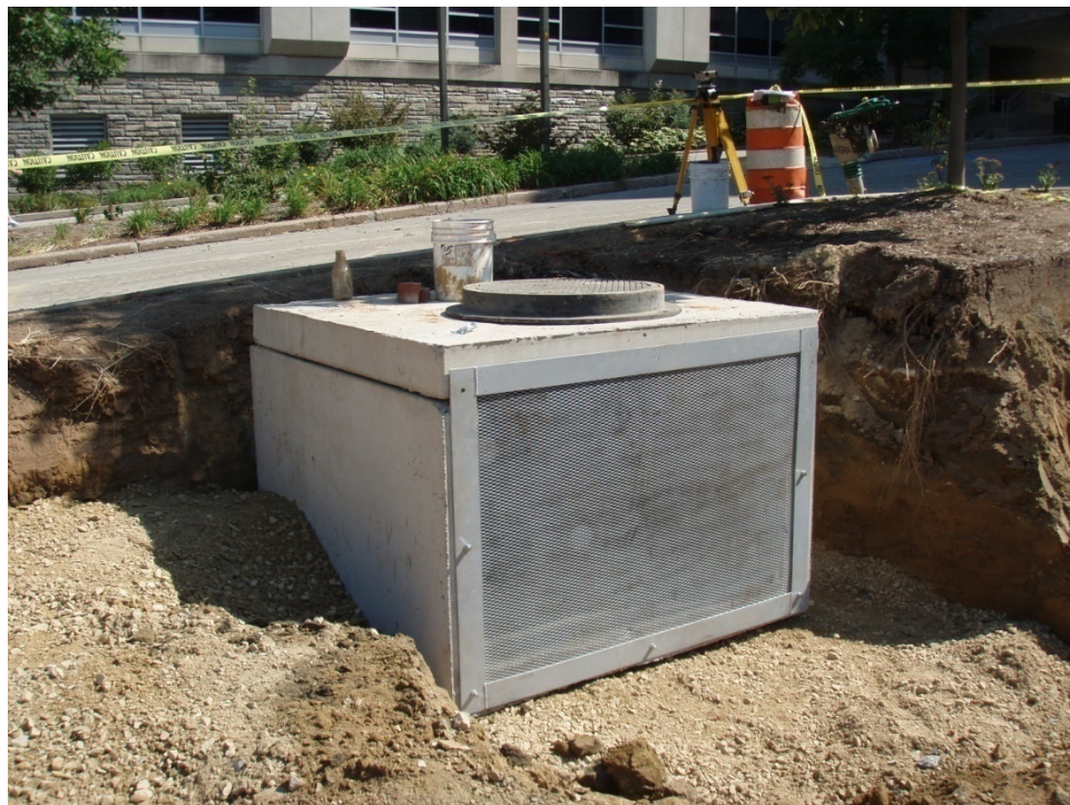
Figure 3-7 Observation Manholes
