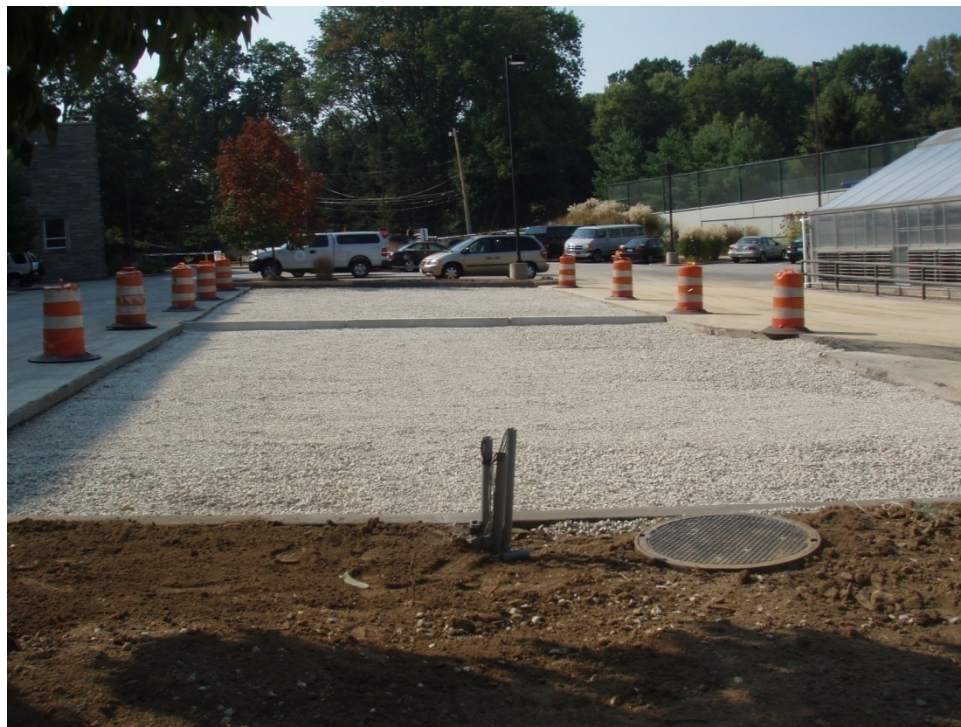
Figure 4-3 Infiltration Bed Filled With Stone
