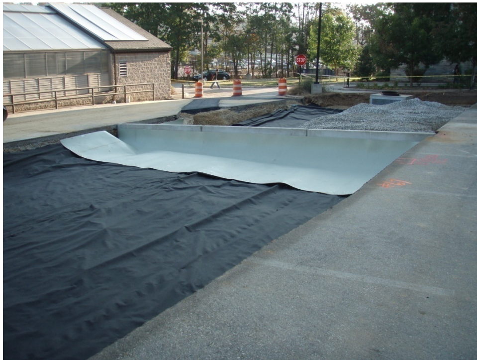
Figure 3-3 Geomembrane (Gray), Geotextile (Black), and Jersey Barrier (Beneath Geomembrane)
