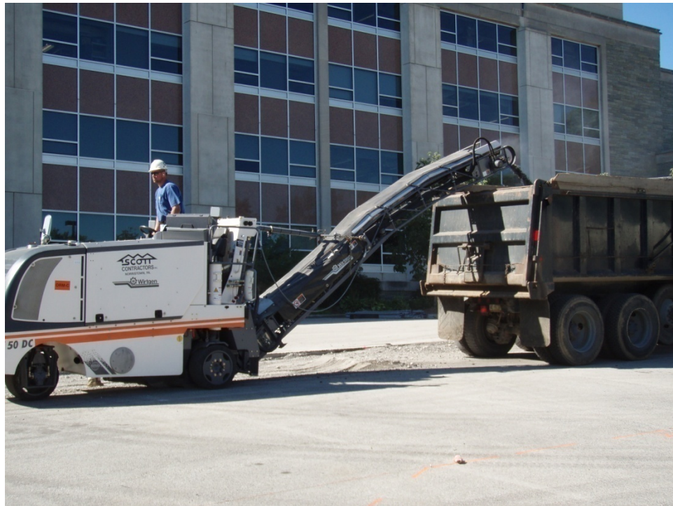
Figure 4-1 Existing Pavement Demolition
