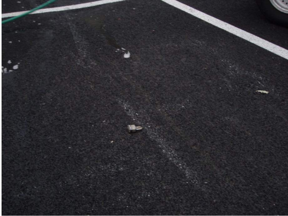
Figure 5-1 Plow Marks on Porous Asphalt
