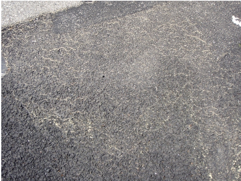
Figure 5-6 Clogged Porous Asphalt
