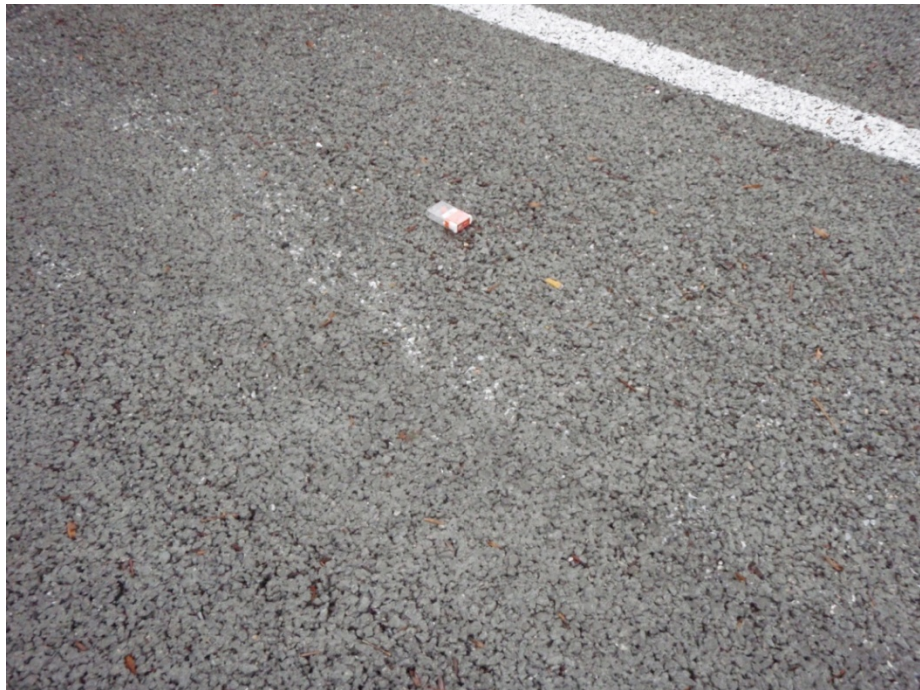
Figure 5-2 Plow Marks on Pervious Concrete
