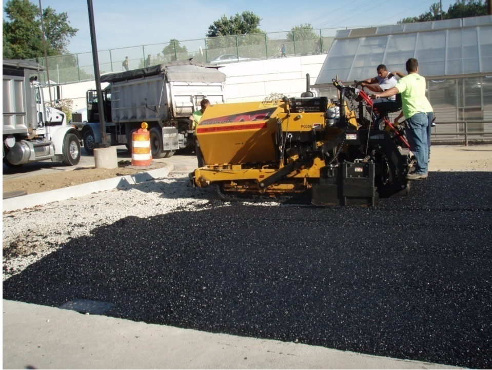
Figure 4-4 Porous Asphalt Installation Using Asphalt Paver
