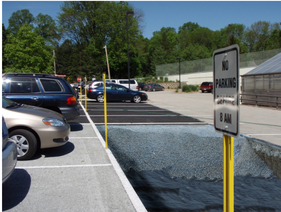
Figure 1-2 Composite Photograph of Porous Pavement Section (porous asphalt in background, pervious concrete in foreground, stone bed and geotextile beneath)
