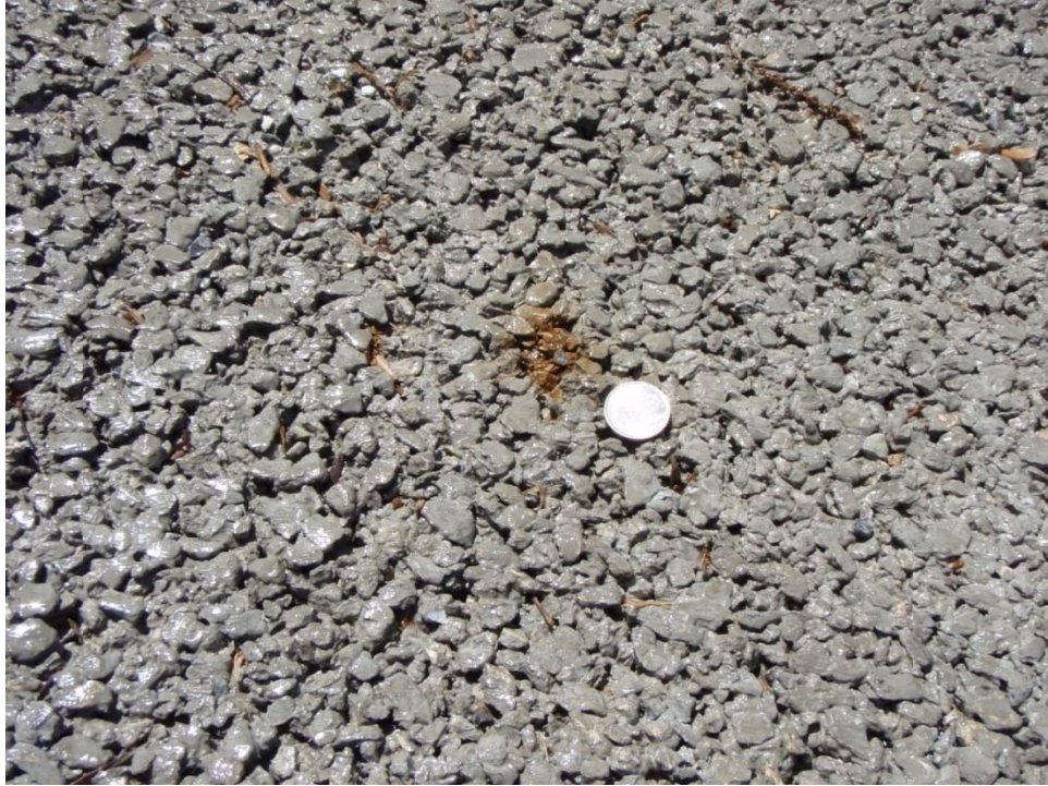
Figure 5-8 Oil Spot on Pervious Concrete
