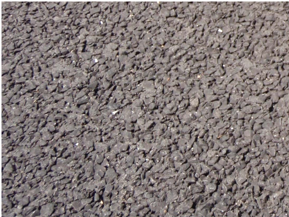
Figure 5-4 Original Pervious Concrete
