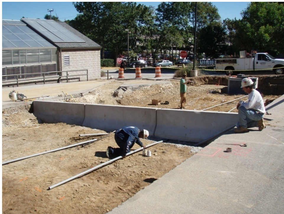
Figure 4-2 Jersey Barrier & Instrumentation Conduit
