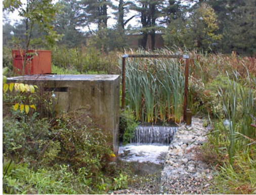
Figure 3.7: Outlet Structure
