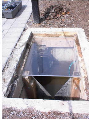
Figure 8.3 Weir located at the Pervious Concrete Outlet
