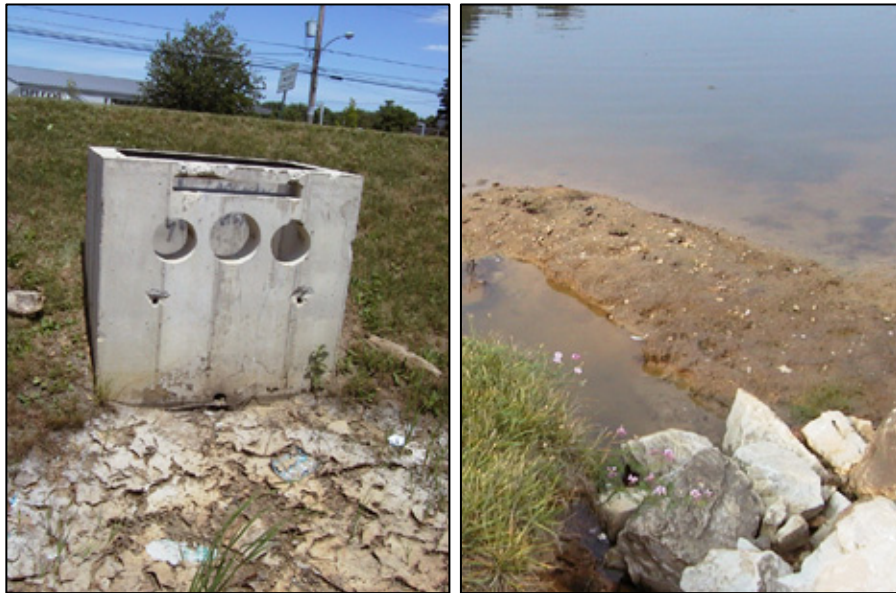
Figure 11. Sedimentation occurring in two detention basins in Chester County, PA.
