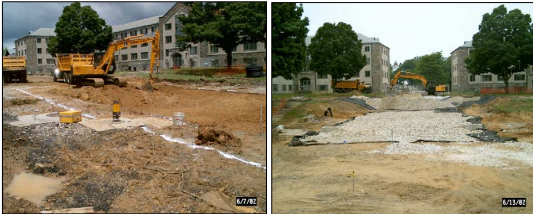
Figure 2. Excavation of the lower bed (left) and placement of the middle bed crushed stone (right).
