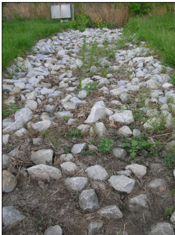
Figure 63. Approximately six years of sediment build-up in a riprap swale at the BTI (photo taken on May 16 th 2007).
