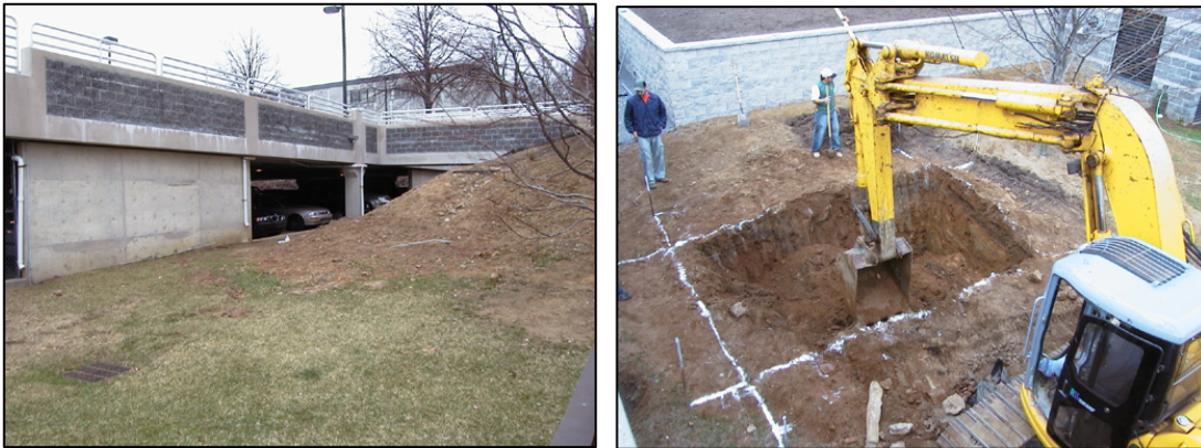
Figure 7. Preconstruction view of BMP location (left) and BMP excavation with retaining wall in place.
