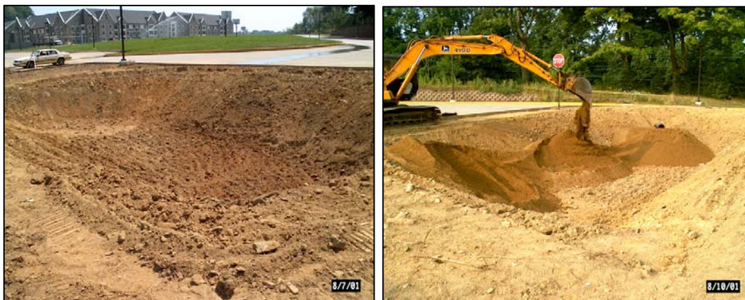
Figure 3. Fully excavated original soil (left) and composite soil placement process (right).
