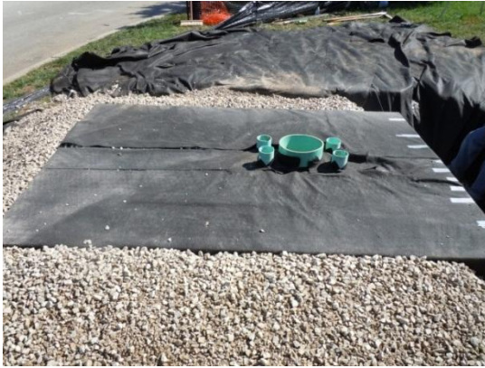
Figure 3.18 - Infiltration trench before topsoil
