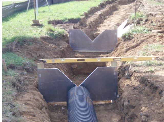
Figure 3.6 - Leveling of weir plates during construction
