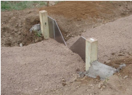
Figure 3.20 - Weir plate installed with concrete
