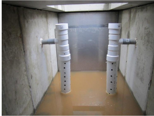
Figure 3.3 - Conduits inside the weir box which exit and turn toward the parking garage
