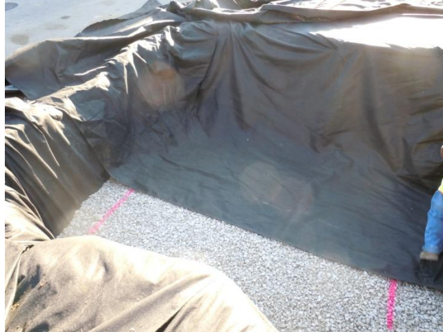
Figure 3.11 - Infiltration trench layers of stone and geotextile before inserting R-Tanks
