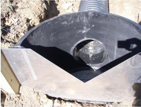
Figure 3.12 - Transition piece following 2nd rain garden
