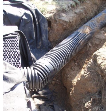
Figure 3.13 - Pipe going into IT
