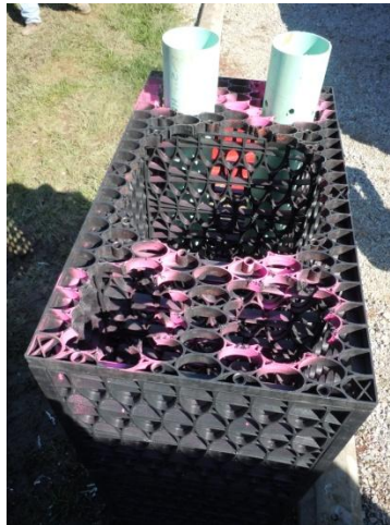
Figure 3.15 - Installation of 4 in PVC in center R-Tank for instrumentation
