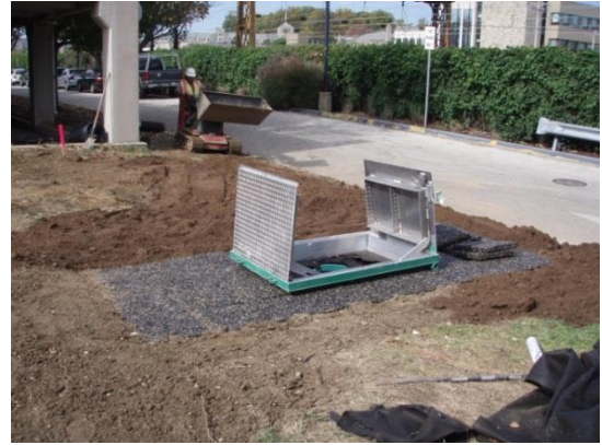
Figure 3.19 - Infiltration trench near completion
