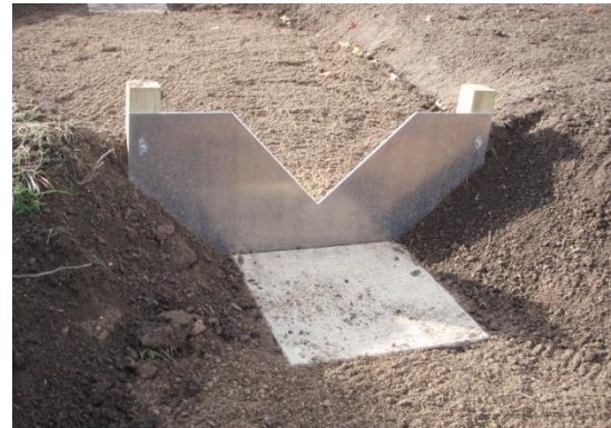
Figure 3.21 – Example of splash pads used to prevent erosion
