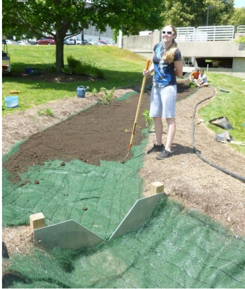
Figure 3.26 - Erosion control mat with topsoil along the swale
