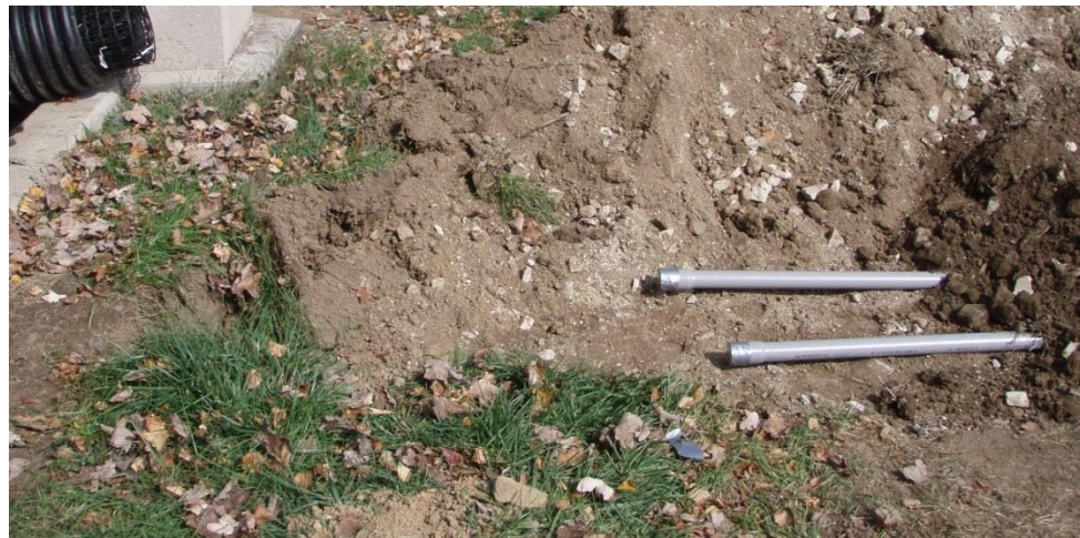
Figure 3.16 - Tee fittings which allow conduit to exit IT
