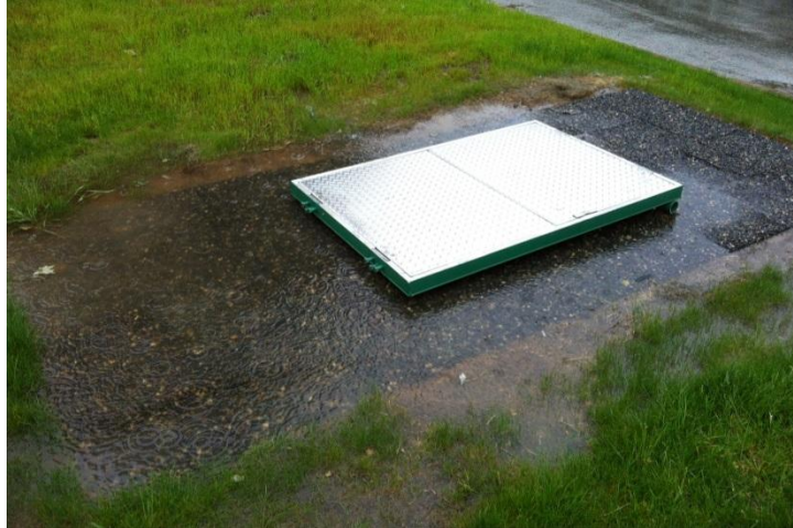
Figure 4.11 - Ponding and runoff on the pervious pavers at the IT (May 2012)
