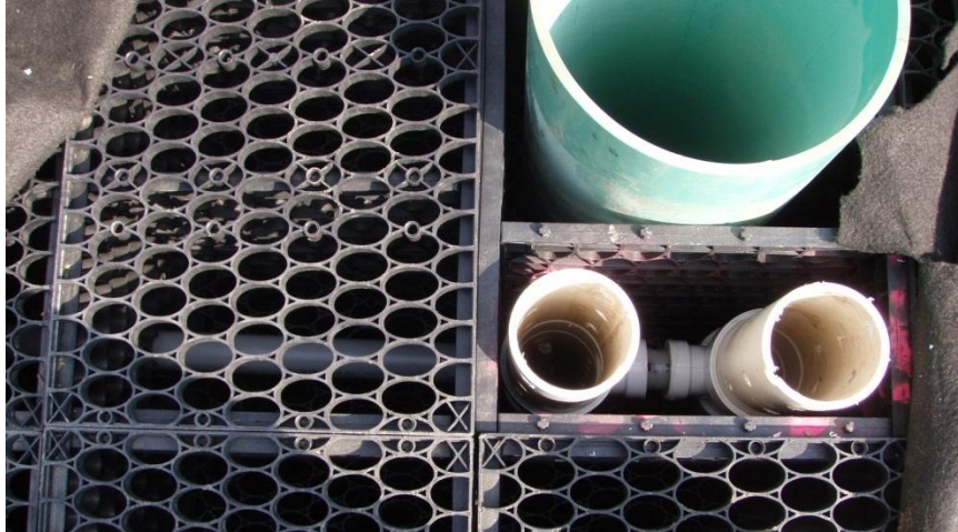
Figure 3.16 - Tee fittings which allow conduit to exit IT
