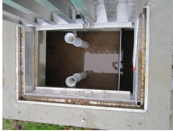
Figure 3.25 - Inside weir box – perforated pipes and second baffle plate
