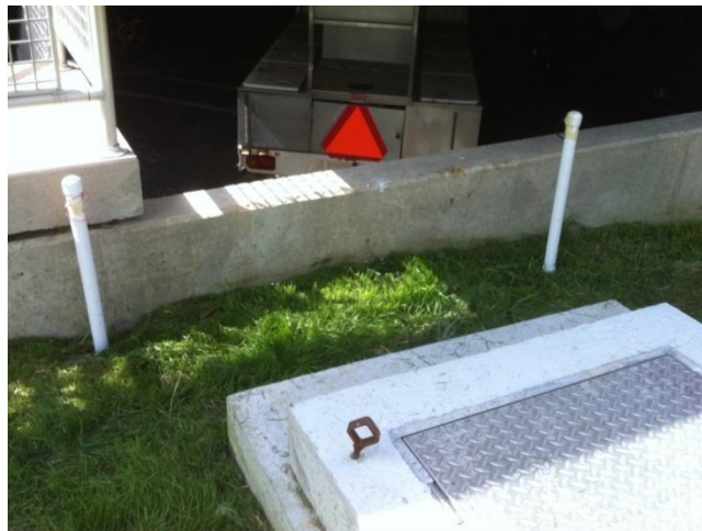
Figure 3.4 - Conduits reaching the garage
