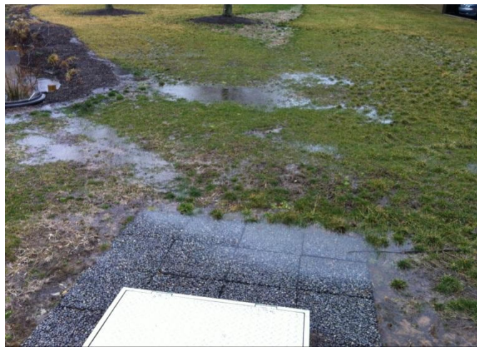
Figure 5.18 - Ponding on the pervious pavers at the IT after a March 12, 2013 storm event
