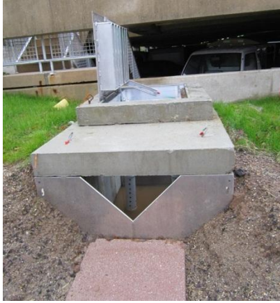
Figure 3.24 - Weir box completed – outflow end with weir plate and splash pad
