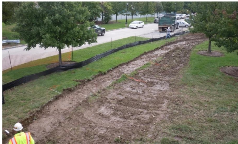
Figure 3.10 - Stripping of topsoil day one of construction
