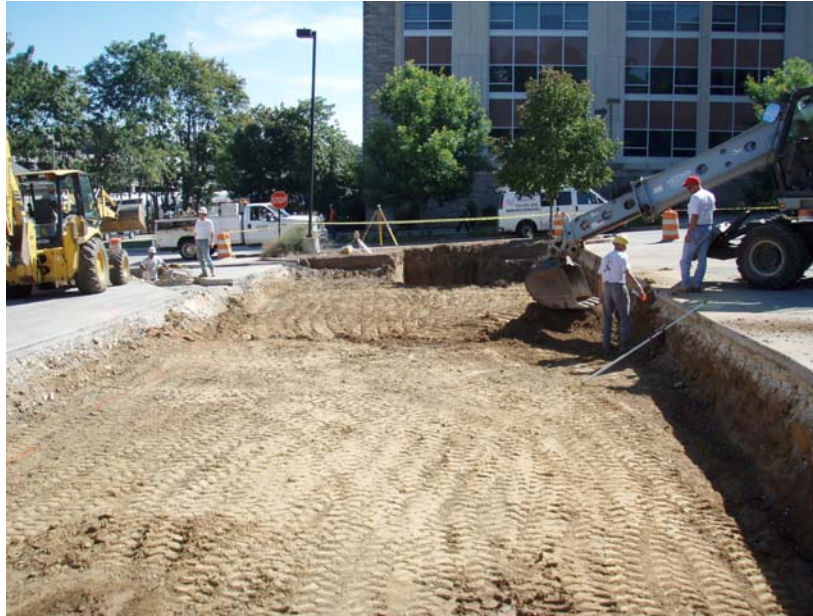
Figure 1.5: Excavation of infiltration beds
