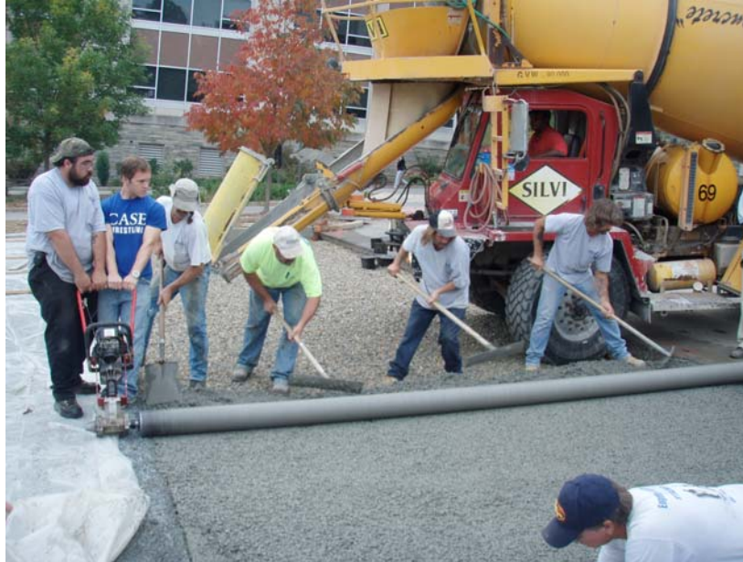
Figure 1.13: Installation of pervious concrete
