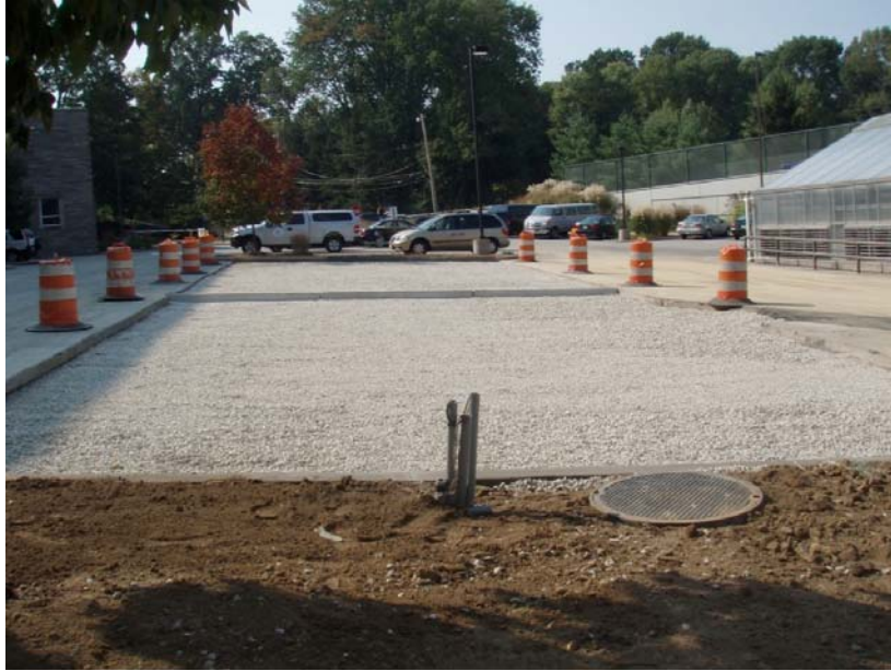
Figure 1.9: Completed infiltration bed filled with clean, washed #2 stone.
