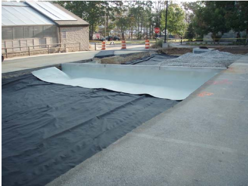
Figure 1.8: Excavated infiltration bed with the jersey barrier (middle) covered by the impermeable membrane (grey) and the non-woven geotextile (black)
