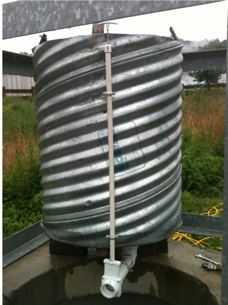
Figure 3.7: Valve and Handle Configuration
