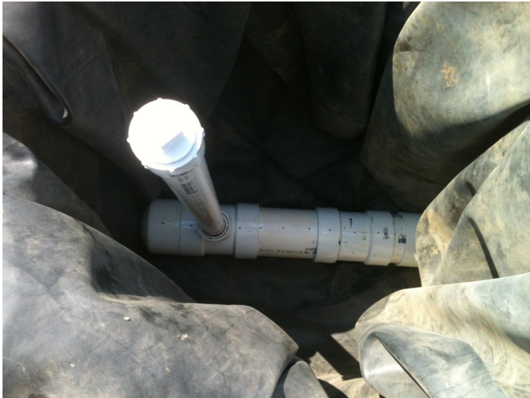
Figure 3.8: Liner and Clean Out Pipe Installation
