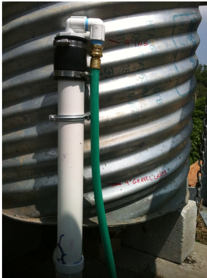
Figure 3.11: Upturned Elbow with Hose Attachment
