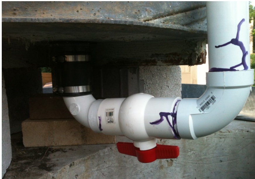
Figure 3.10: Upturned Elbow with Valve
